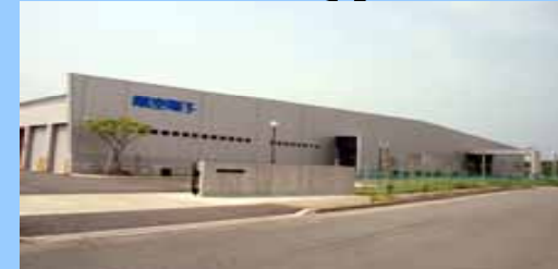
Adding a new factory building
