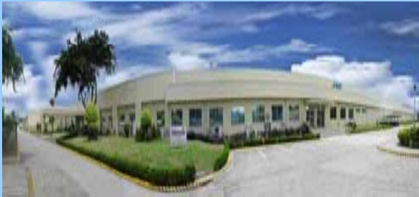
Construction of a second plant
