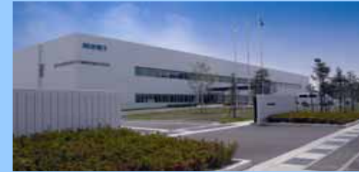
Adding a new factory building
