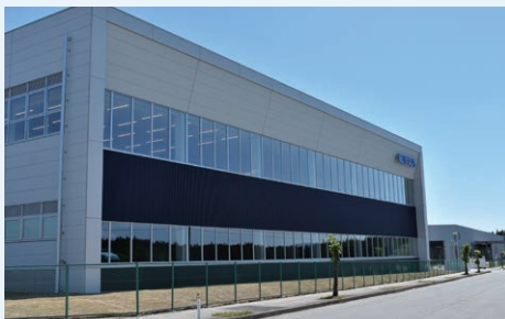
2nd Plant B Building, JAE Yamagata (completed in May 2023)
