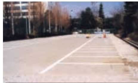
Underground storm water infiltration basin (completed)
