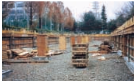
Underground storm water infiltration basin (under construction)
